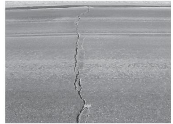
Thermal Cracking (Low Temperature)
