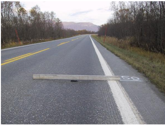
Rutting (High Temperature)
