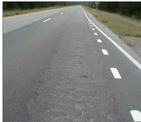
Fatigue Cracking (Intermediate Temperature)
